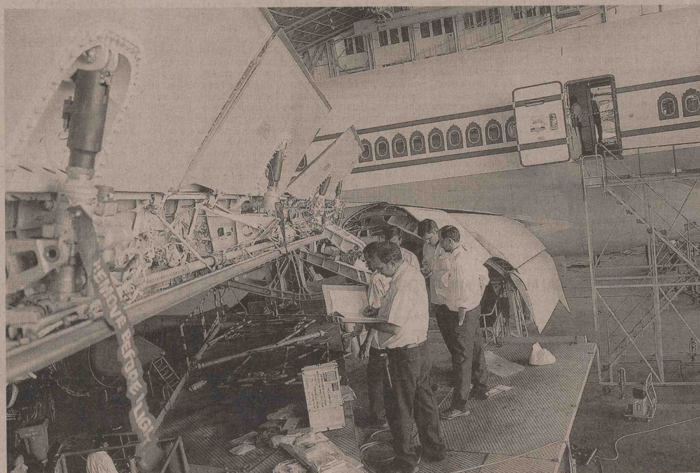
Workers carry out maintenance operations at an Air India facility
